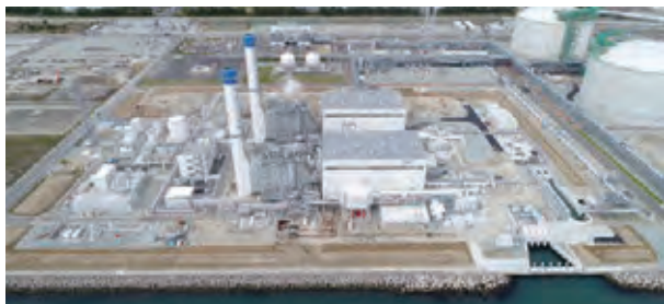
Fukushima Natural Gas Power Plant
