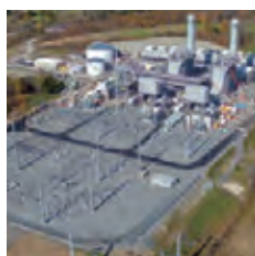
Fairview Natural Gas-Fired Thermal Power Plant in the United States
