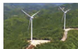
Inami Wind Power Plant
