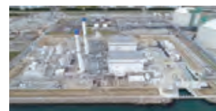
Overall view of the power plant
