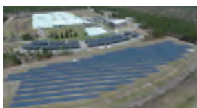
Solar power plant developed and constructed by SolAmerica Energy, LLC in USA Courtesy of SolAmerica Energy, LLC
