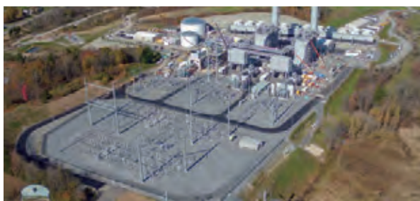
Fairview natural gas-fired thermal power plant in the United States
