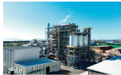
Hirohata Biomass Power Plant (Hyogo Prefecture)
