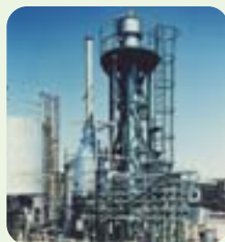
Wet Catalyst Oxidation Process Plant
