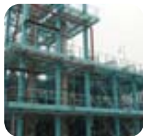
Petrochemical wastewater treatment plant (under construction)
