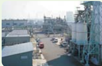
Torishima Carbon Material Center
