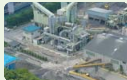
Excavation Soil Recycling Plant
