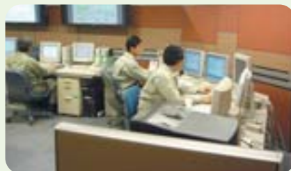
Cogeneration remote monitoring center
