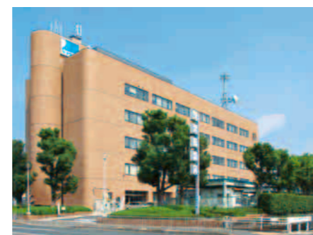
Hokubu Gas Building (Takatsuki City, Osaka Prefecture)
