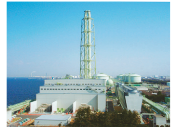
Senboku Natural Gas Power Plant (Takaishi City, Osaka Prefecture)
