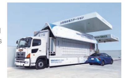
Kamitoba Hydrogen Station
