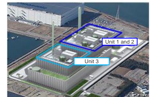
Himeji Natural Gas Power Plant (Rendering, including Unit 1 and 2 under construction, and Unit 3 in planning)
