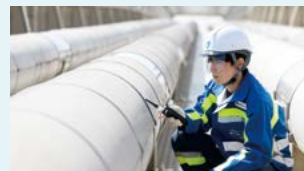
Regular inspection of gas pipes on bridges
