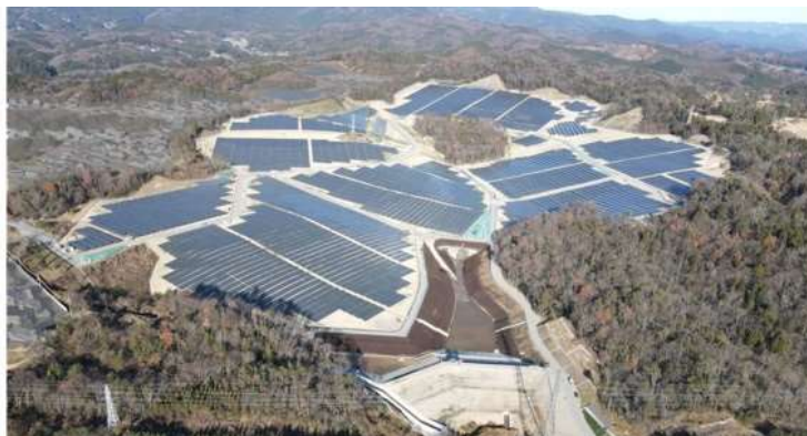
Figure-6 Isohara Extra-high Power Plant
