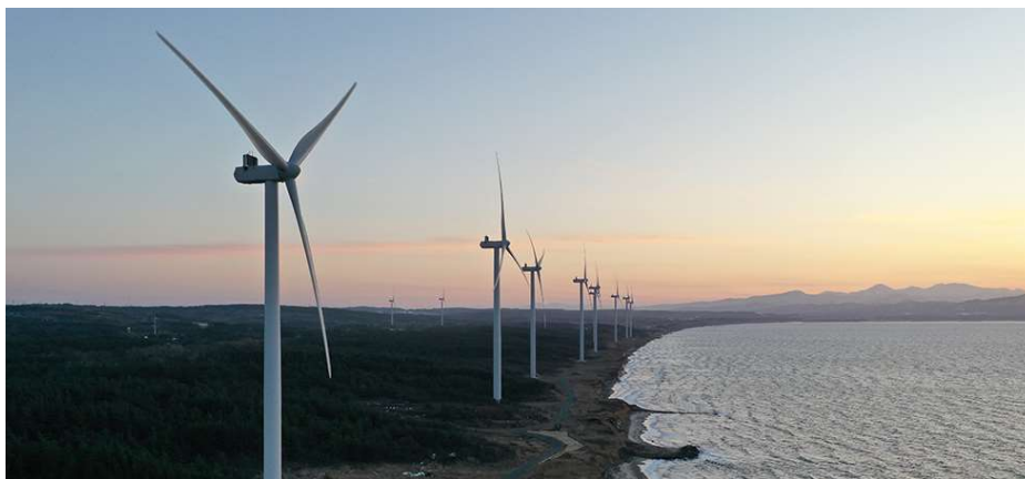
Figure-3 Noheji Mutsu Bay Wind Farm
