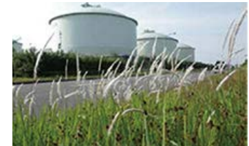
Green belt planted with Cogon Grass at Senboku LNG Terminal
