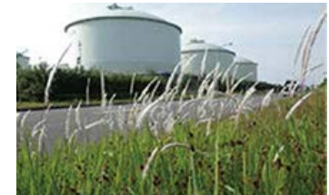
Green belt planted with Cogon Grass at Senboku LNG Terminal
